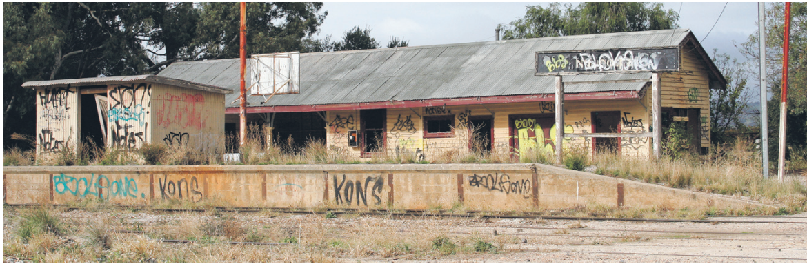
The once-bustling Nuriootpa Railway Station is set to be demolished.
